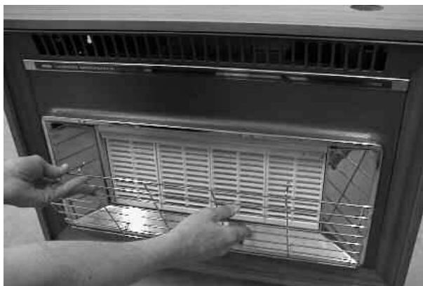
Fig. 2 Remove the Dress Guard.
